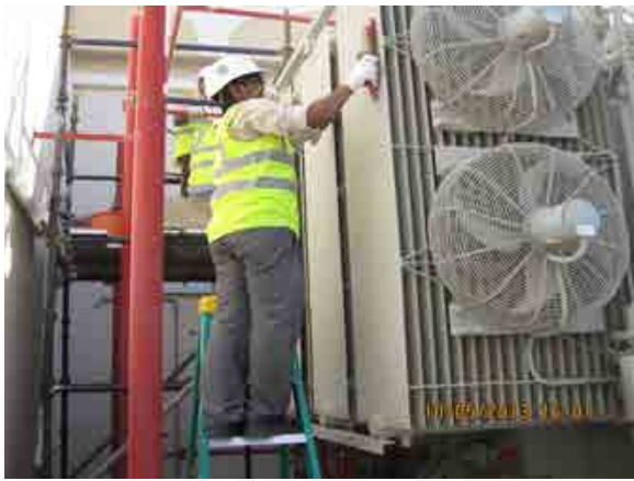
Schedule maintenance of Sub-station
