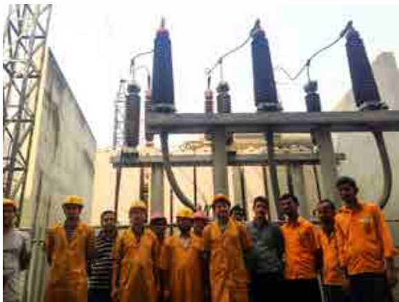
Schedule maintenance of Sub-station at Gulshan Area
